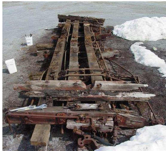
In the end, none of the original car body's wood was salvageable. So, now the team had to documentate the remains of the car and then carefully removed all the metal parts so they can be used on the new carbody.
