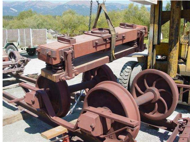
Lowering a rebuilt truck bolsters into place on the rebuilt frame.
